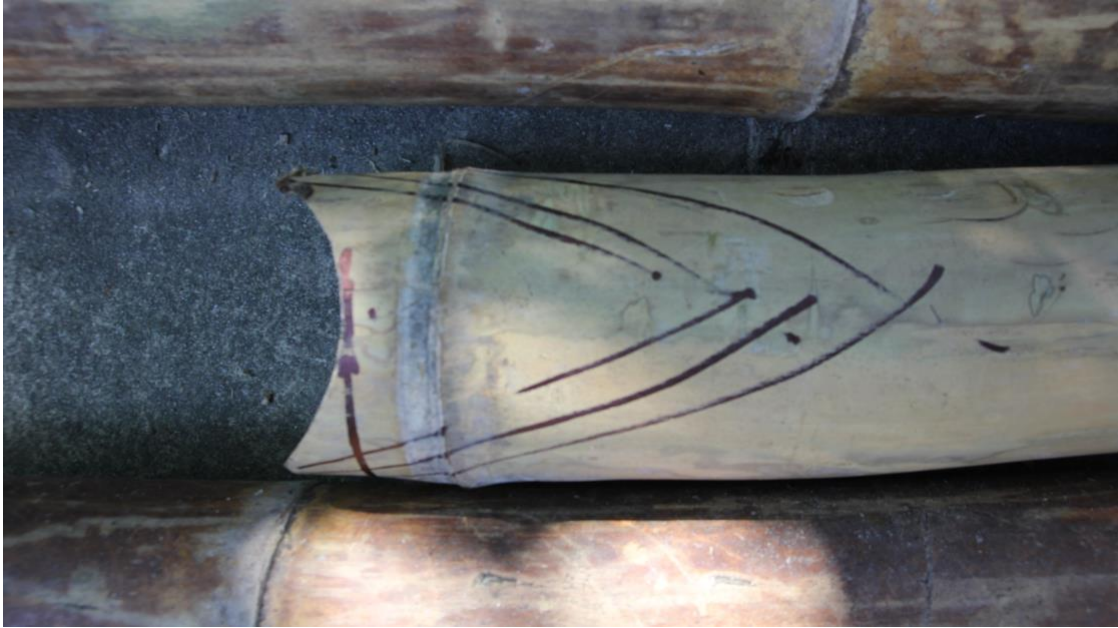
Figure 14 – Markings and adjustments made by the traditional craftsmen – levels of accuracy and geometrical control.
