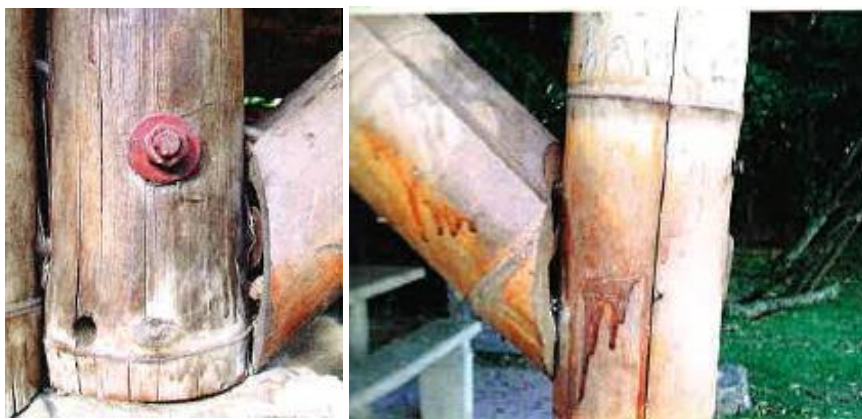
Figure 8 - Images showing typical bad workmanship in cutting the bamboo to couple with the receiving bamboo – Source: Building With Bamboo – Gernot Minke
