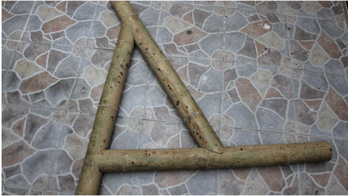
Figure 13 – Image of a digitally fabricated reciprocal triangulated connection.
