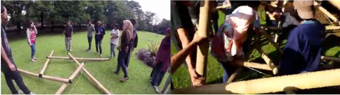
Fig. 8. Initial process and lowest member pre-tensioning
