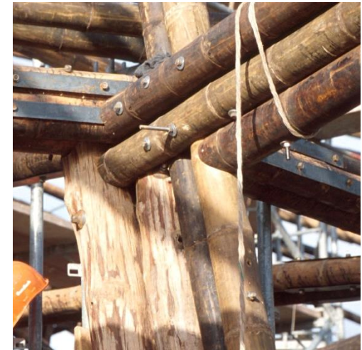
Joint detail. ZERI pavilion. 2000
