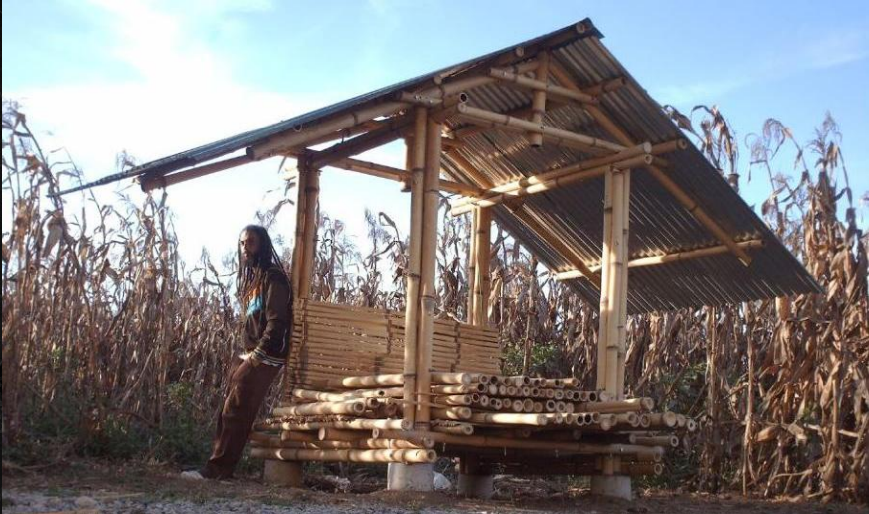
- Construction of Bamboo Drying Shed -
