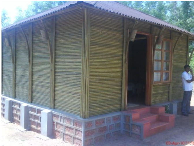
Model Bamboo Hut at Kudal 2010 (KONBAC) erected with CCB treated bamboo (A good example of realizing potential of bamboo)
