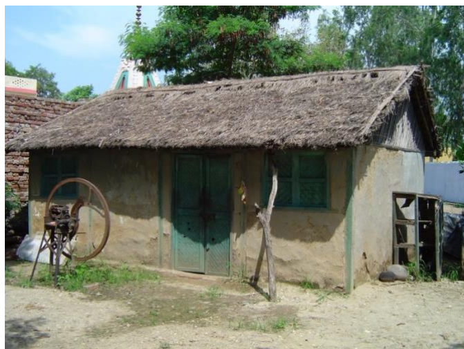
Fig.7. Treated bamboo reinforced Mud hut (constructed 1983)after 24 years service (Picture taken 2007).
