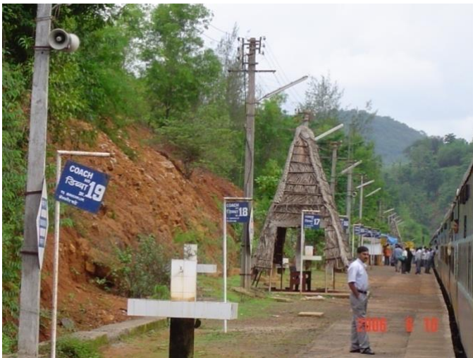
Bamboo and thatch used to make passenger shed on Konkon Railway
