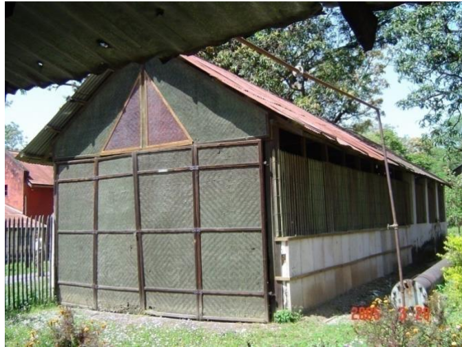
Fig.3. Air seasoning shed for wood/Storage Shed (FRI) using CCA treated bamboo mats for shutters and split bamboo reinforced mud walls (Year erected 1957; Picture taken in 2006).
