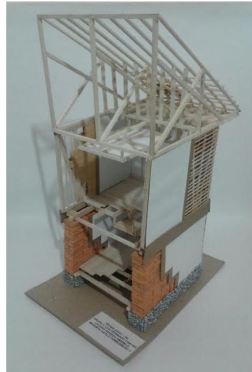
3- MAMPOSTERIA LADRILLO BAHAREQUE DE TIERRA BRICK MASONRY CLAY BAHAREQUE
