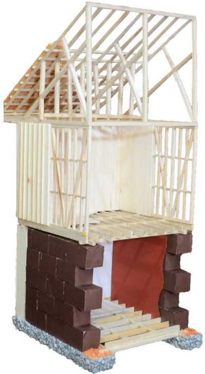
4- MAMPOSTERIA LADRILLO BAHAREQUE DE TABLA BRICK MASONRY TIMBER BOARD BAHAREQUE
