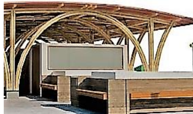
Centro Comercial – tubulares en fibra de bambú guadua Shopping Center – tubulars in bamboo guadua fiber Filandia, Quindío
