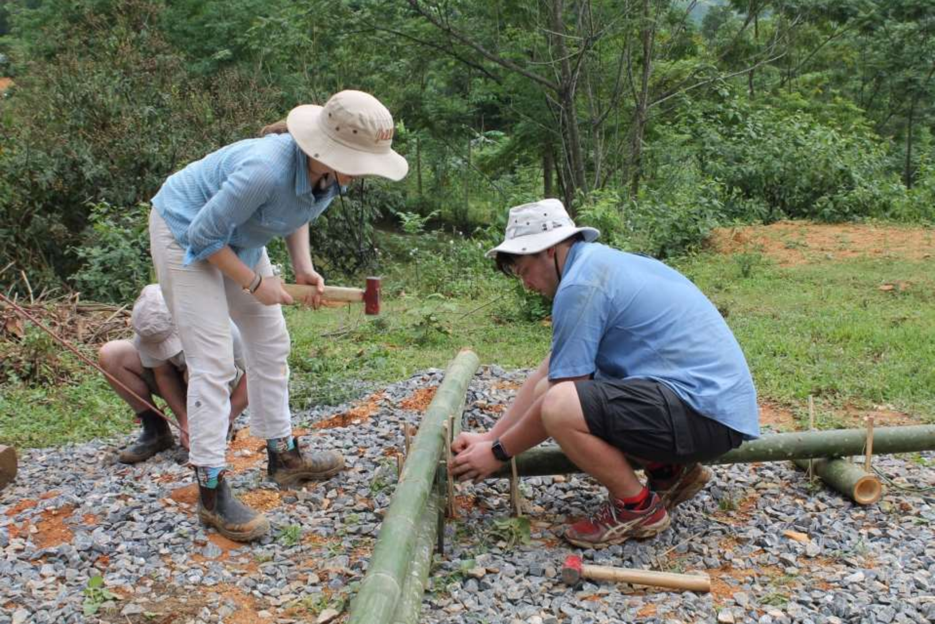
Bamboo dowels were used to set up a jig so that all four frames to be constructed to the same profile.
