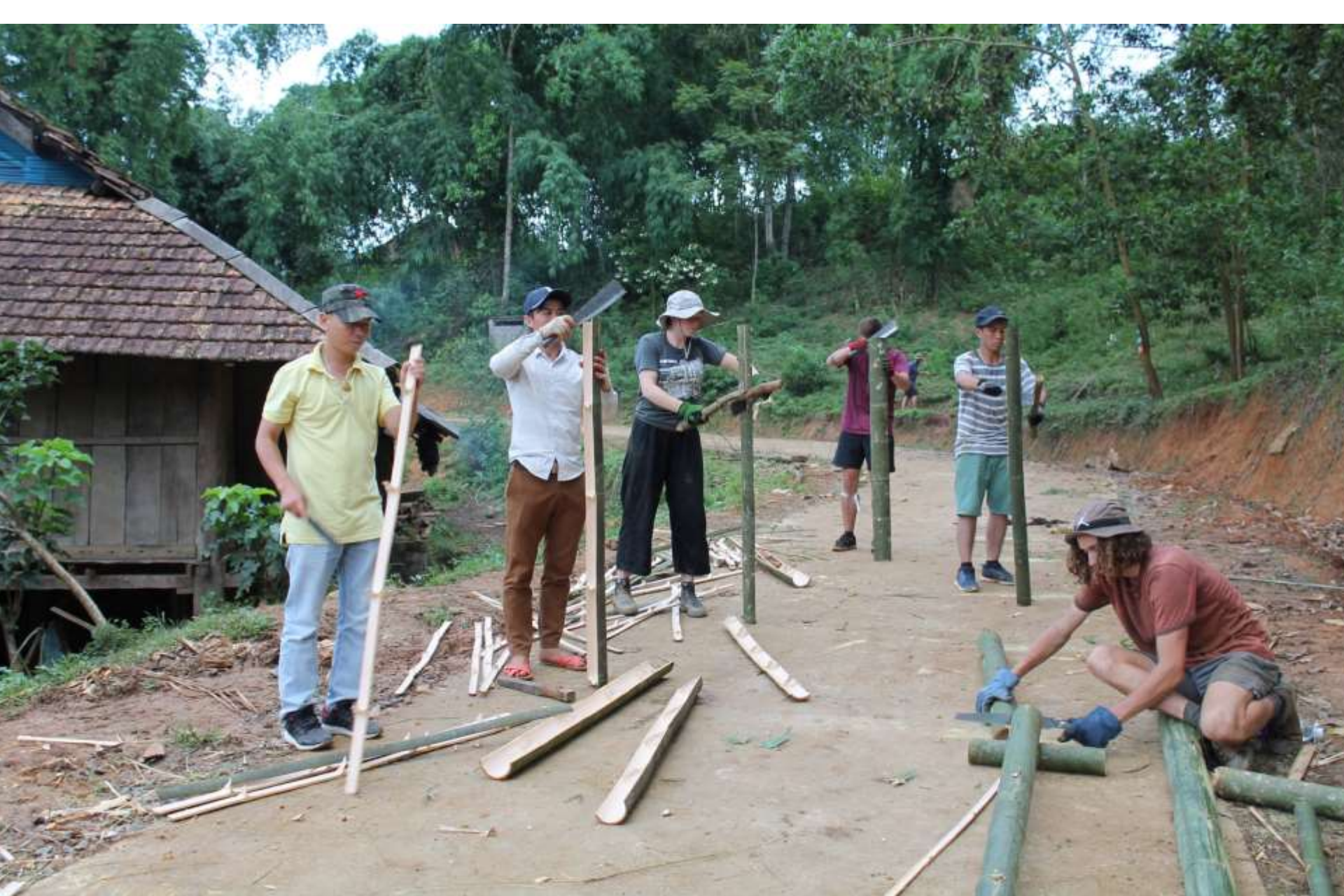
Throughout the building process, a constant split factory continued along the road. Lengths of bamboo were cut to site and split down their length.
