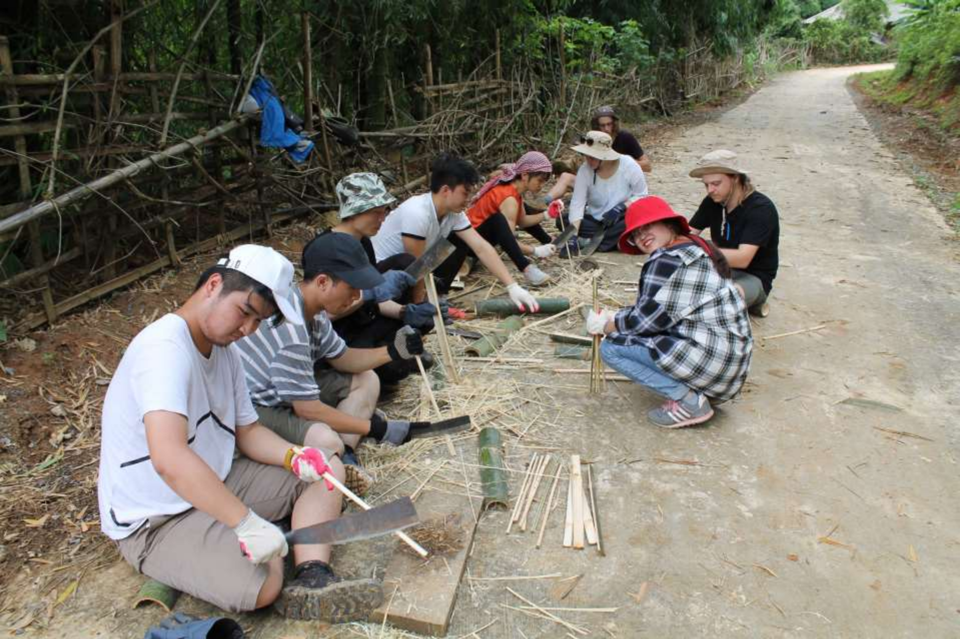
Production of bamboo pins to be used for joining bamboo structure.
