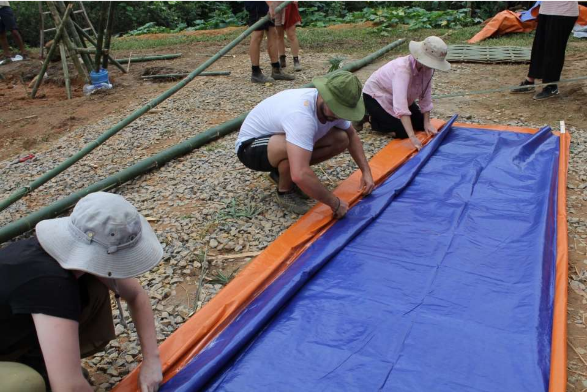
Tarpaulins, which are employed for a range of different uses, were used as the lining for the roof
