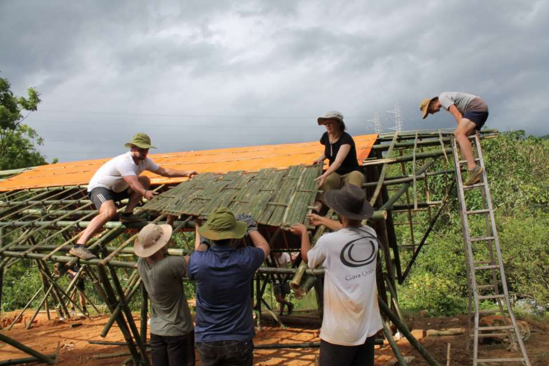
The 1.5m x 1.5m roof panels were passed up on to the roof...
