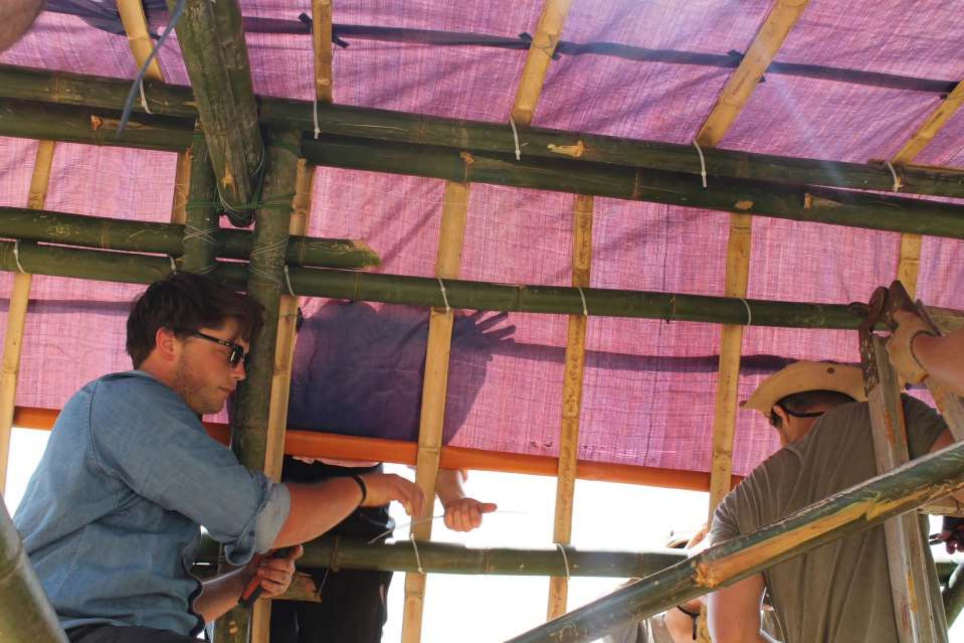
Teams worked above and below the structure, feeding the wires through the tarp and then fixing underneath.
