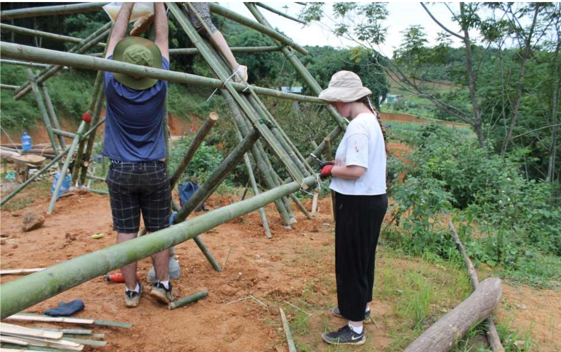
Bamboo splits were used to form battens, which span across the purlins, to support the roof tarp.
