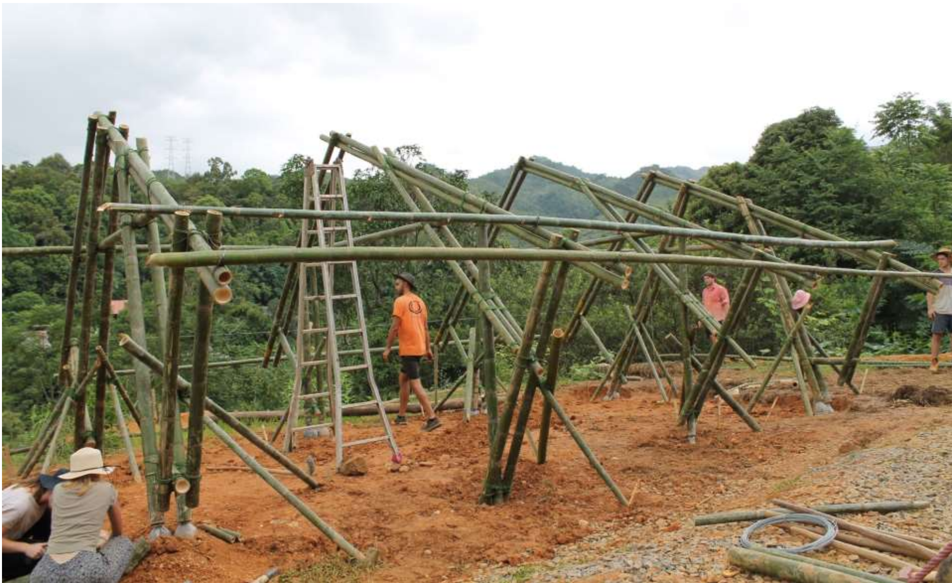
The portals were lashed together with bamboo poles...
