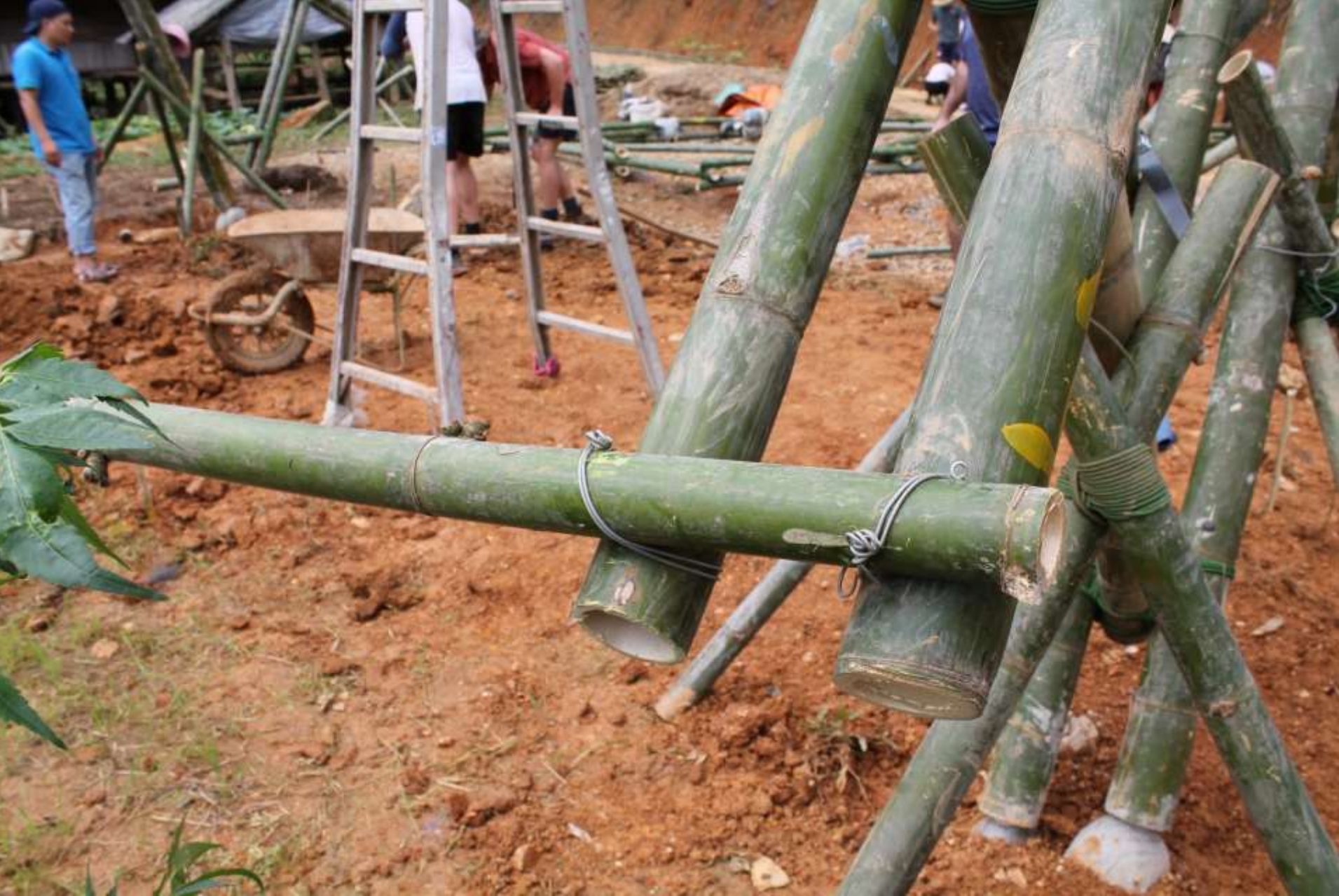
Wire was used to join the battens to the frame...
