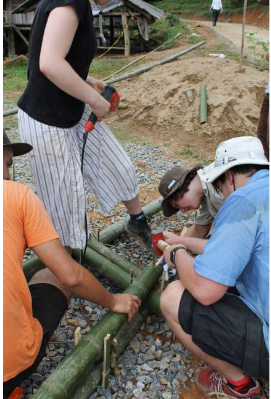
The first of many holes were drilled and pinned with bamboo dowels, and the building process commenced.
