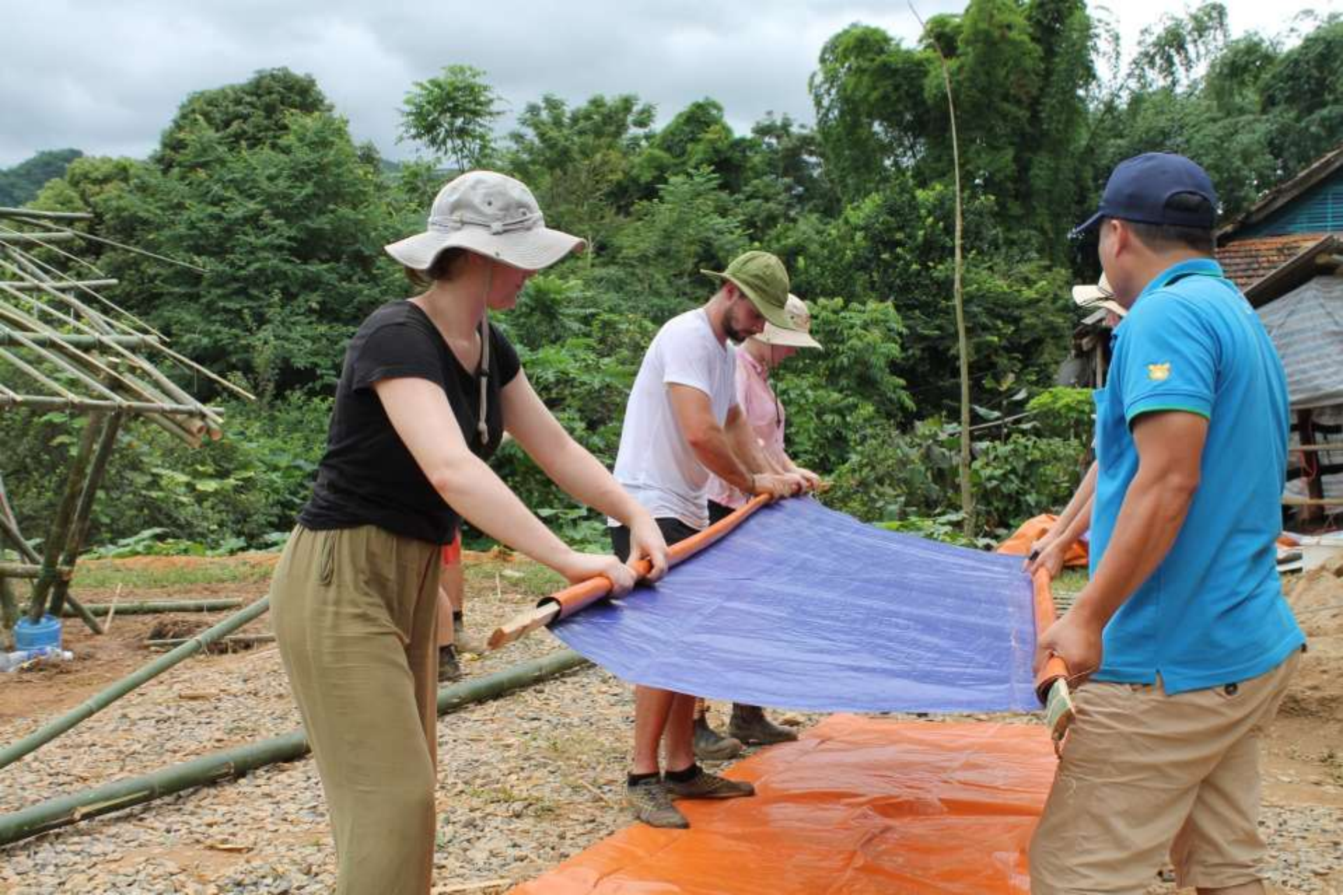
Bamboo splits were folded and rolled into the tarps for ease of handling.
