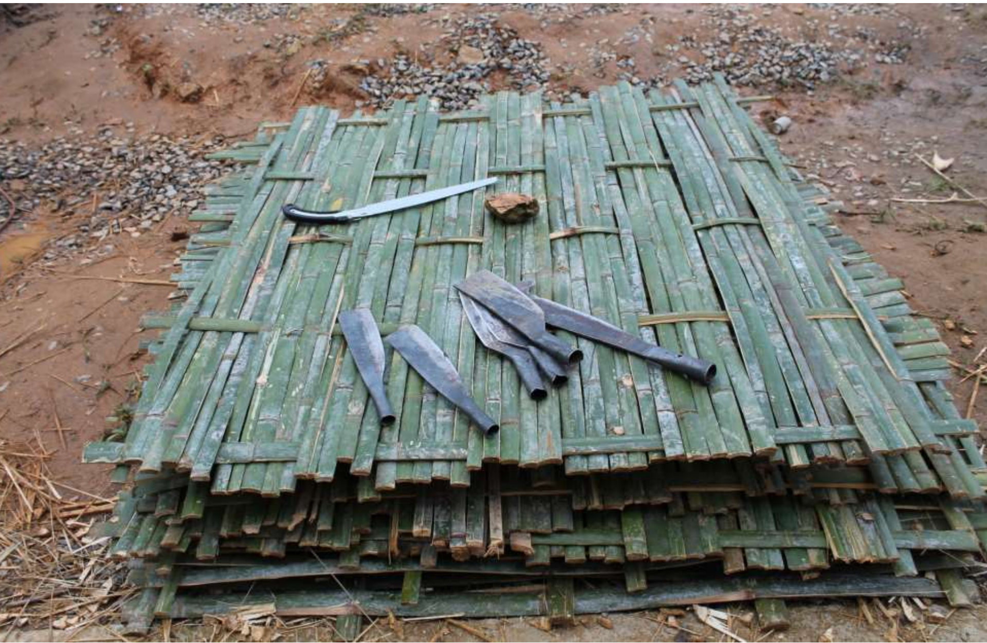
Roof panels were prefabricated...
