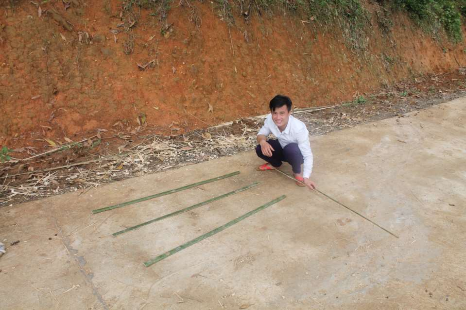
Bamboo set out to in place to form the weft...
