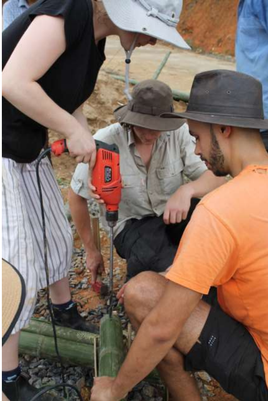
The first of many holes were drilled and pinned with bamboo dowels, and the building process commenced.
