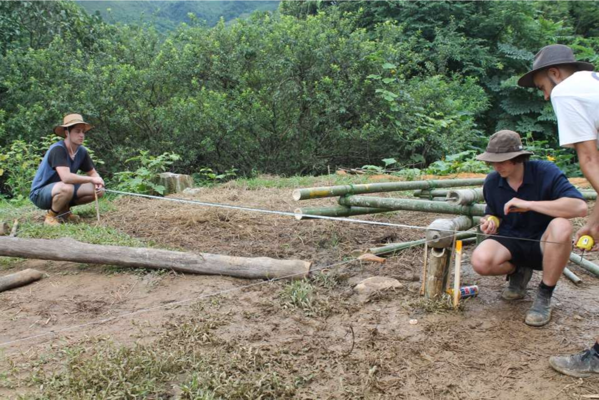
A structural grid was laid out over the site to locate the position of the portals.
