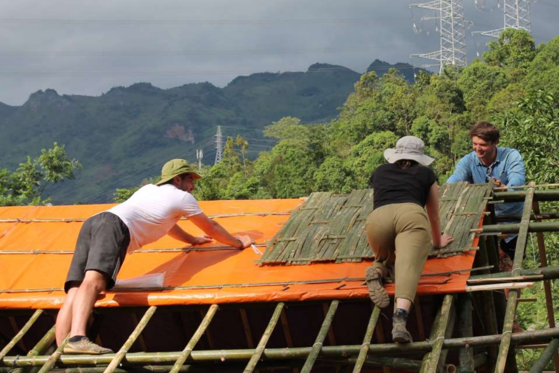
The 1.5m x 1.5m roof panels were passed up on to the roof and fixed to the battens...
