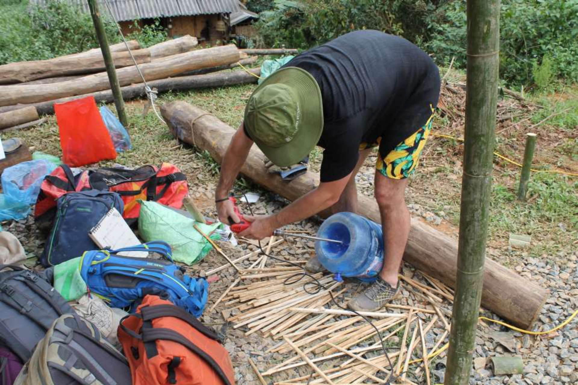
Larger bottles were used for the single poles of the structure.
