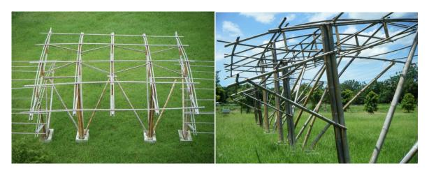
The first year of bamboo studio opened in 2009. Students are to develop a simple structure on campus using the method of prefabrication. They decided to create a small pavilion next to the Rugby field. The design of roof frames were influenced by the geometry of a rugby football.
