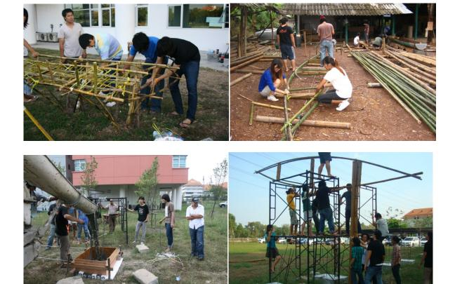
During semester, students had to create mock-up models for structural test. After the design is done, they will learn to do real construction and build pre-assembly parts at off-site, and bring to site to put together the final product.
