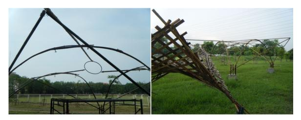
The second year studio also continued to explore the art of bamboo structure in prefabricating assembly. Students created two prototypes of small pavilion that can be installed and taken off by simple tools and man power. The prototype can also be connected with another same kind to create a larger space combined.
