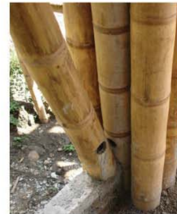
Bracing with Guadua culms
